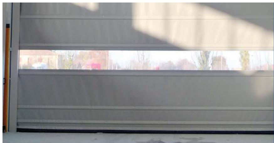
**Struttura:** self-supporting in pre-painted, galvanized or stainless steel sheet
